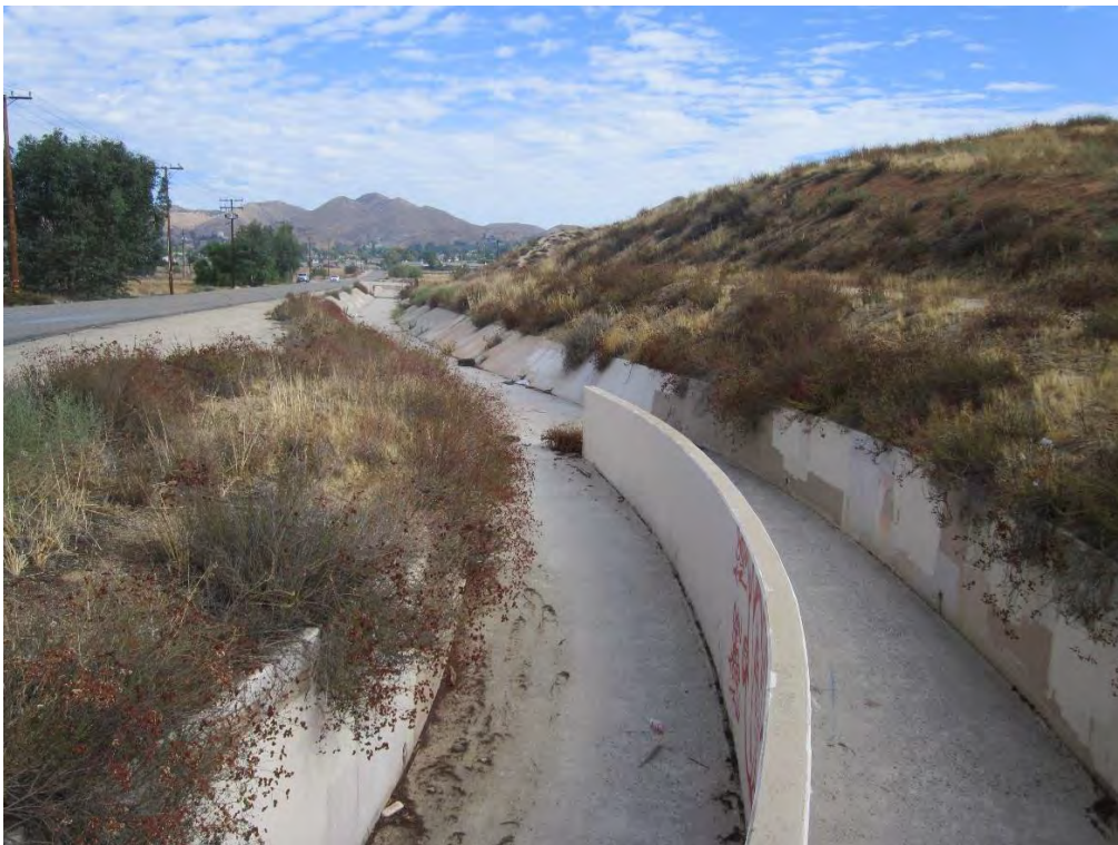
Figure 5. Overview, Linear Segment at Monte Vista Drive, View north, September 12, 2017, Photo #850
