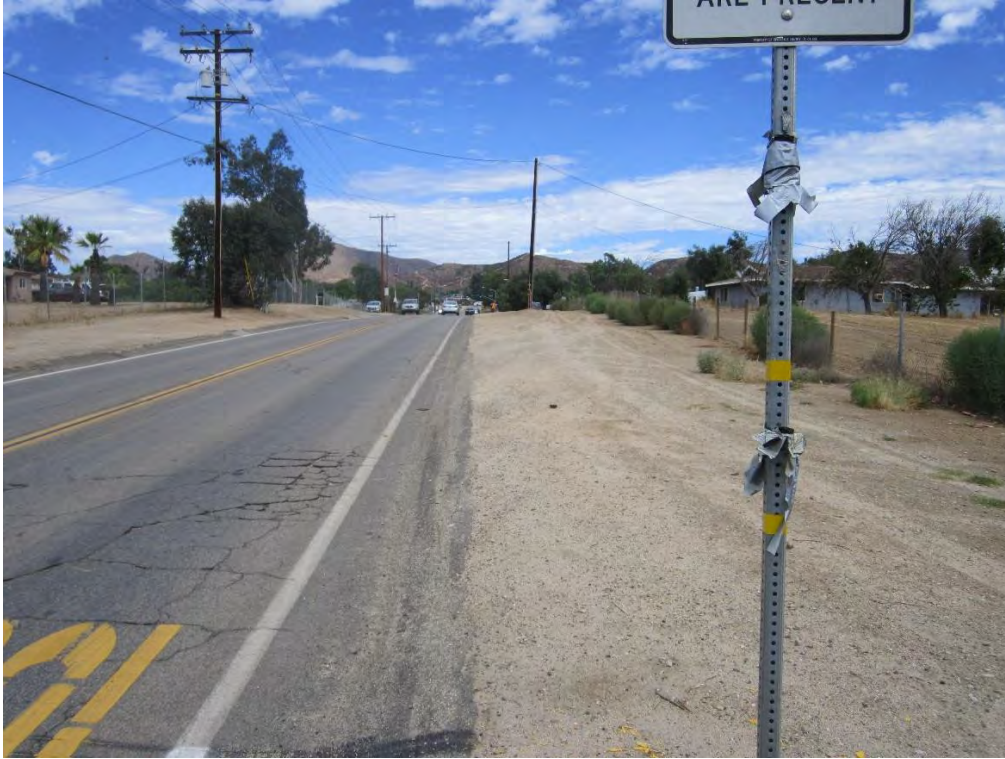
Figure 6. Overview, Linear Segment at Central Street, View north, September 12, 2017, Photo #862
